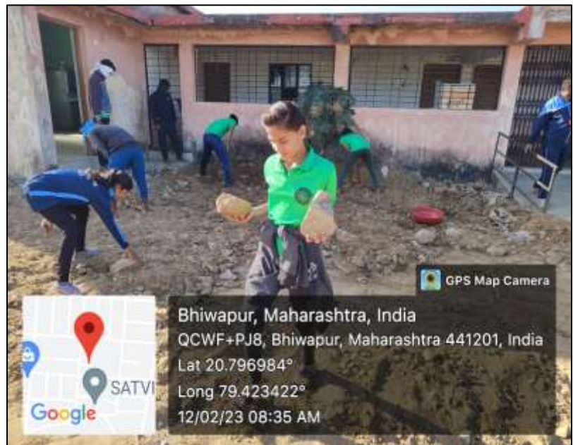
The Volunteers of N.S.S., in action, during the 'Shramdaan'
